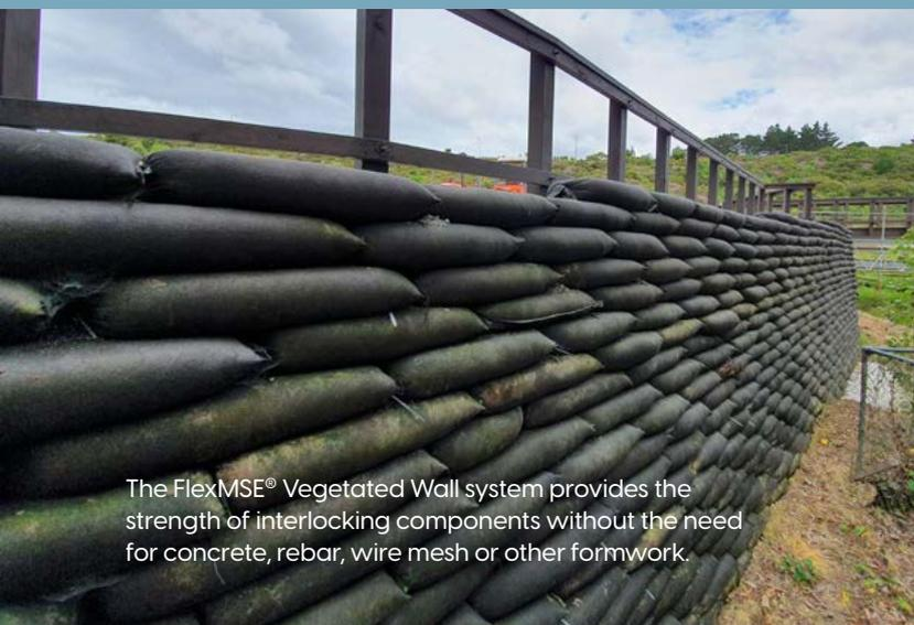
The FlexMSE® Vegetated Wall system provides the strength of interlocking components without the need for concrete, rebar, wire mesh or other formwork.
