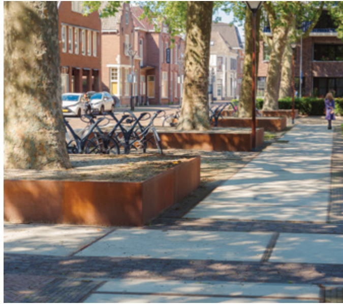
RETAINING WALL CORTEN STEEL
