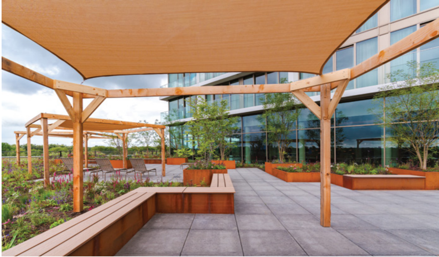
RETAINING WALL BESPOKE
