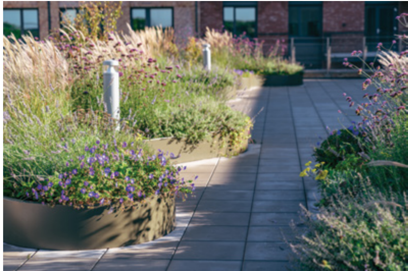
CURVED RETAINING WALL COATED STEEL
